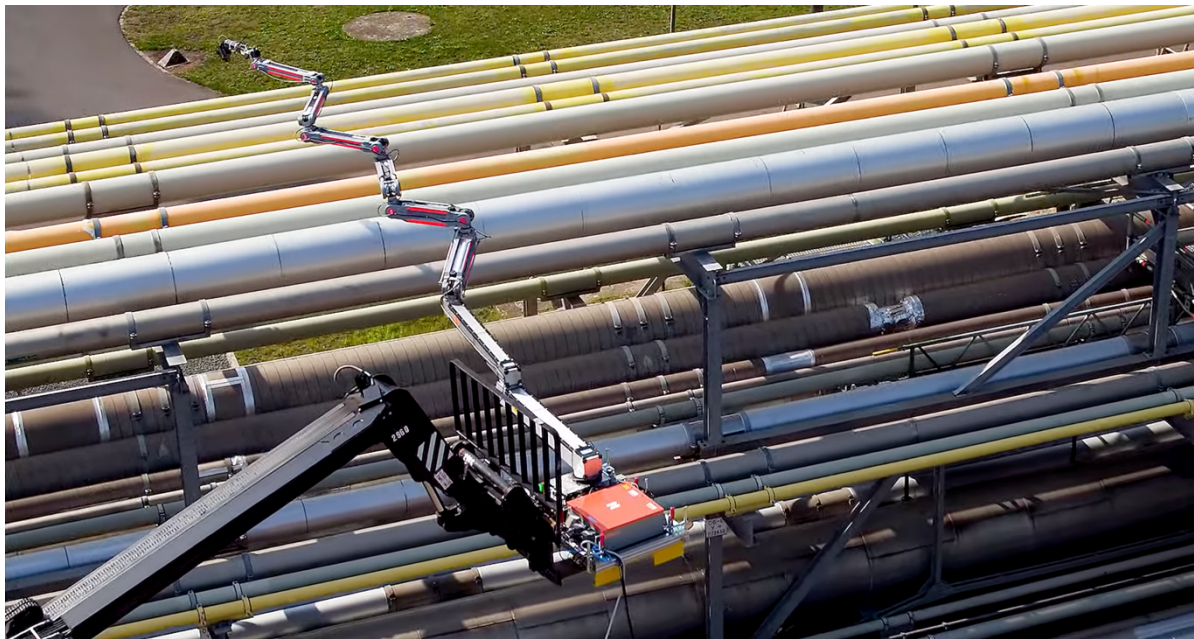
Float Arm during validation tests over pipe racks at BASF Antwerp
